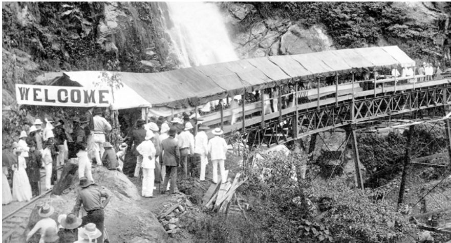
Surveyor Monk was surely present at the opening of the Stoney Creek Bridge. Consisting of four 50ft and three 30ft spans, the bridge was one of the most important on the Kuranda railway. – SLQ APO-025-0001-0010
